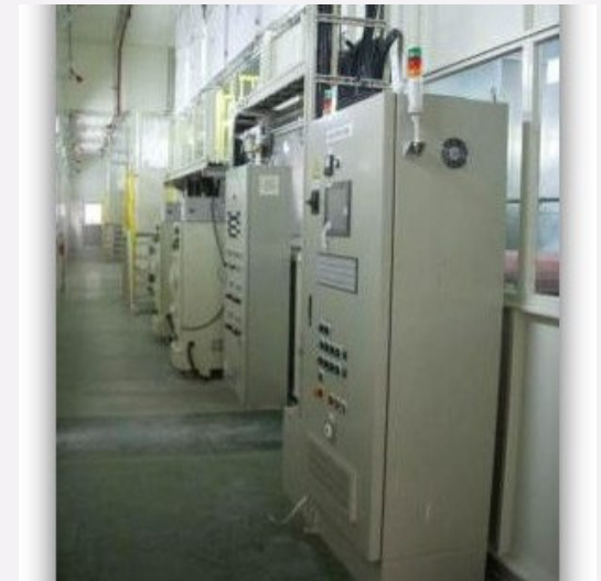
Main Control Panel Installation
