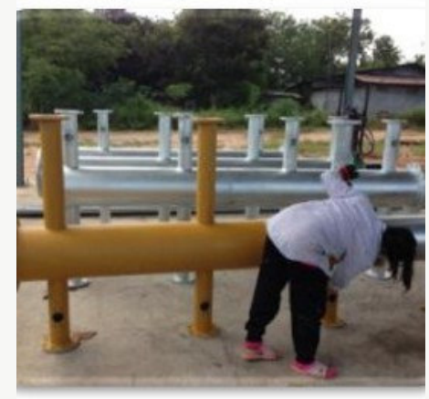
Main pipe Fabrication and Epoxy Coating
